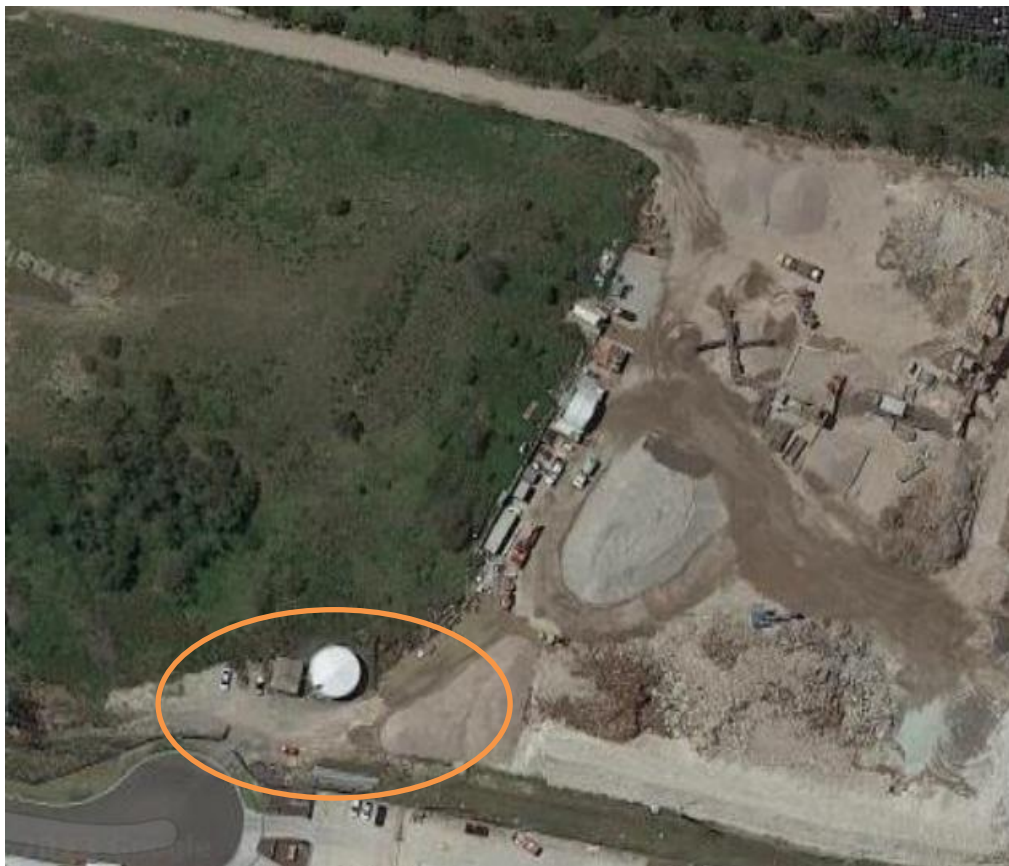
ECORR Rear Yard Workshop Storage Area
